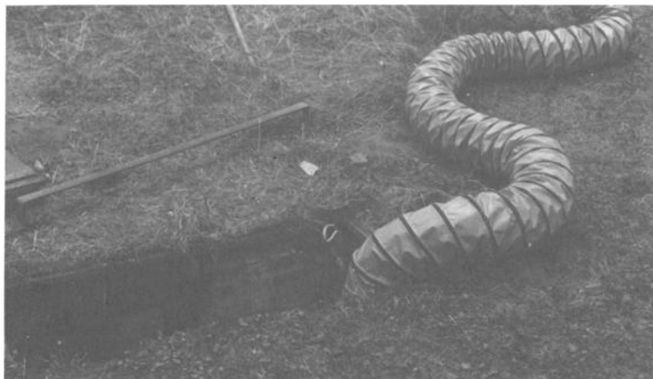
FIG. 3— Demonstration of blower-utilized ventilation of confined space.
